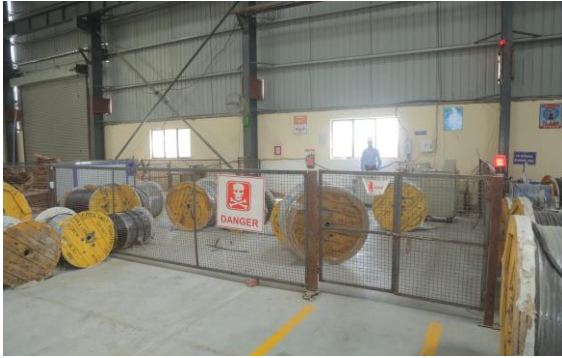
High Voltage Testing Area
